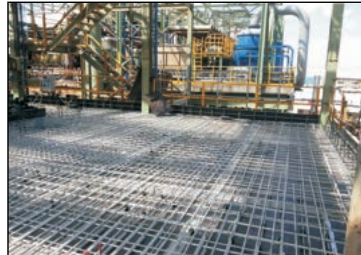
POTASH PLANT CONCRETE SLAB REPLACEMENT GHOR EL SAFI, JORDAN
