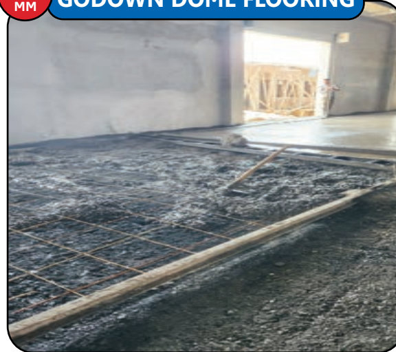
GODOWN DOME FLOORING
