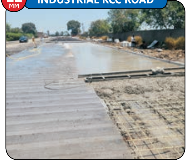
INDUSTRIAL RCC ROAD
