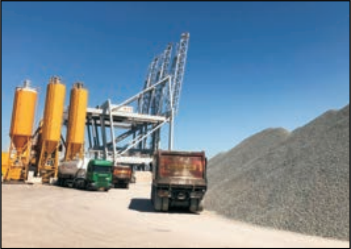
PORT OF ROTTERDAM, NETHERLANDS (CONTAINER TERMINAL UPGRADES)
