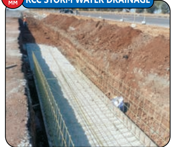
RCC STORM WATER DRAINAGE
