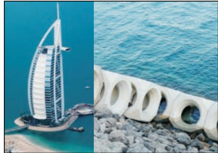
SEAWALL STRENGTHENING THE ICONIC BURJ AL ARAB DUBAI, UAE
