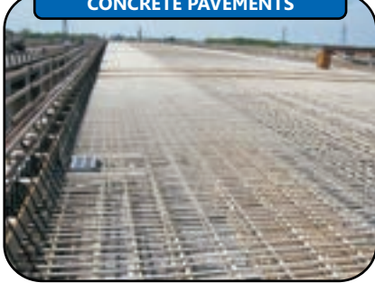
CONTINUOUSLY REINFORCED CONCRETE PAVEMENTS
