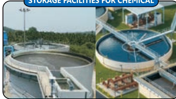
STORAGE FACILITIES FOR CHEMICAL
