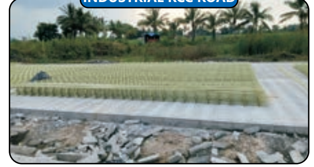
INDUSTRIAL RCC ROAD
