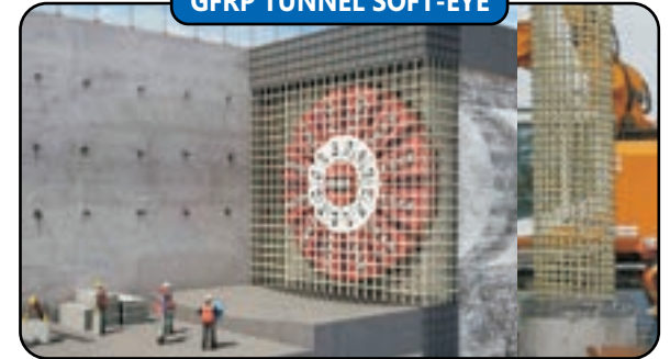
GFRP TUNNEL SOFT-EYE
