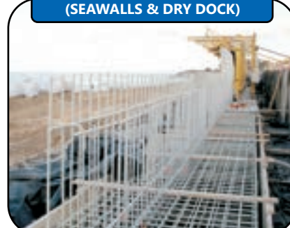
MARINE STRUCTURES (SEAWALLS & DRY DOCK)
