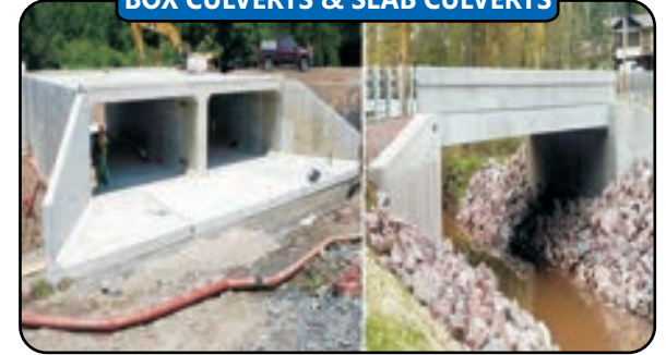
BOX CULVERTS & SLAB CULVERTS
